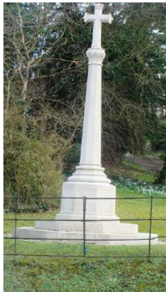
Picture 20. War Memorial well maintained and in good condition.
