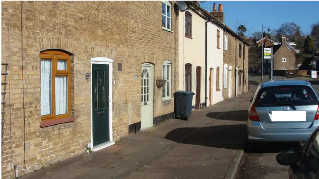
Picture 3. 20-29 Cambridge Road. Terrace of Listed Buildings dating from late 18th century. Whilst doors and windows are in original openings, a more pleasing result would have been achieved had common designs been applied (see picture below).
