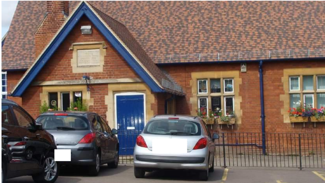
Picture 13. School building Ermine Street. An important component of the Conservation Area both in terms of visual and historic importance. Some fine original features that should be retained.
