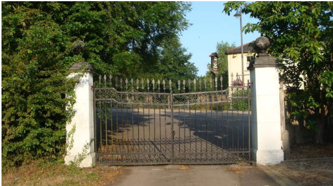
Picture 18. Decorative iron gates and piers on entrance drive to Youngsbury - a grade II* historic Park and Garden.
