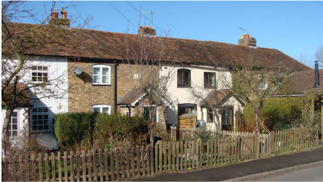
Picture 6. 31 Cambridge Road. The centrally located house with the plaque is listed. Others in the terrace described as having been 'altered' demonstrate the conflicting problems of resolving a good environmental solution to small historic properties versus providing additional accommodation.
