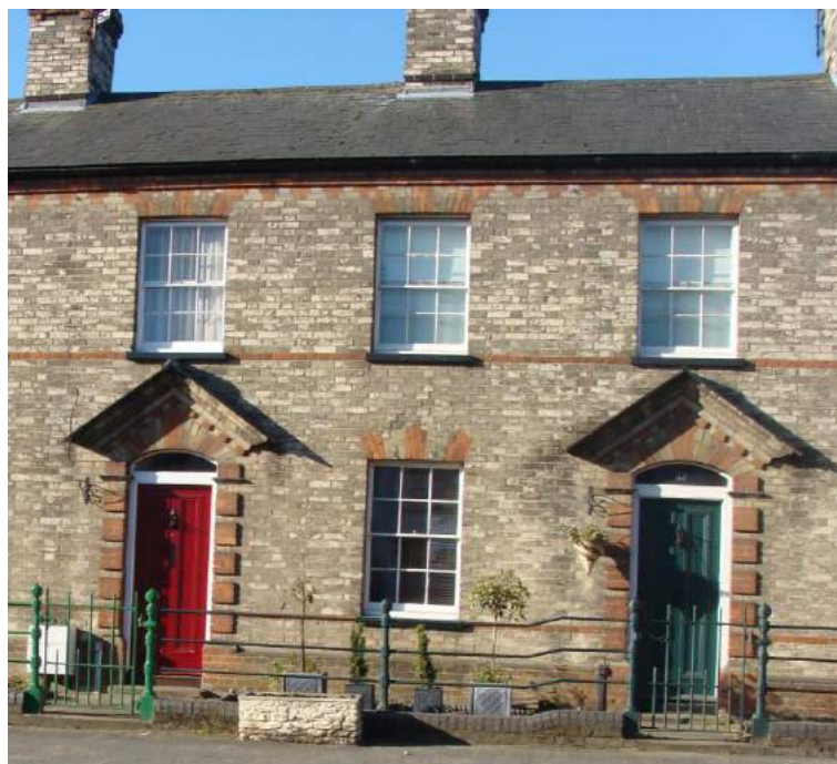
Picture 4. A terrace not local to Thundridge and Wadesmill: the purpose of this photo is to illustrate the importance of design detail. The retention of detail of an historic listed terrace depends on simple repetitive detailing, including original windows and doors. Expression of ownership can be provided by painting doors different colours. Compare with previous picture.
