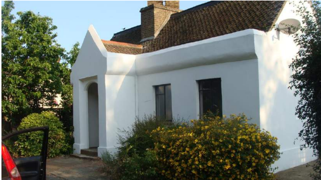
Picture 8. South Lodge - single storey rendered Lodge, tiled roof slate ridge and later metal windows. Whatever its status in law (i.e. curtilage listed or not) it is a building that is worthy of retention.
